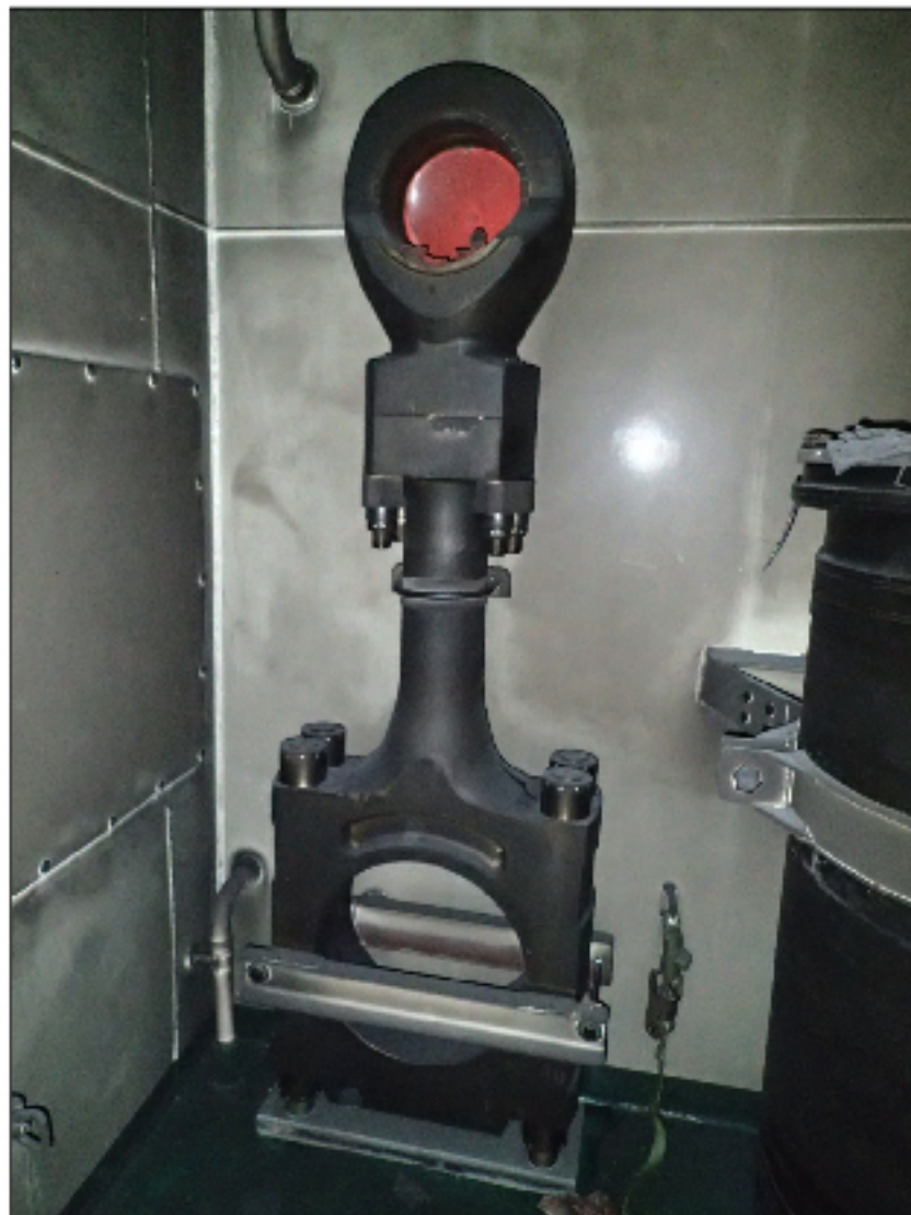
Figure 9: Replacement connecting rod in the THETIS D's engine room
