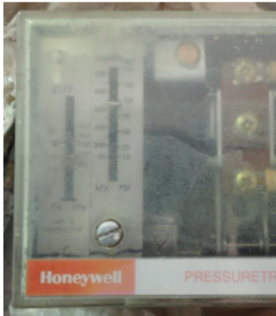
Figure D.36.26 Pressuretrol Controller
