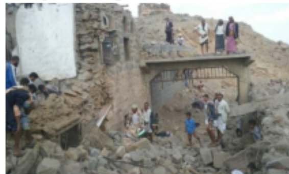
Figure C.58.5 Damage to al-Maqadhi houses
