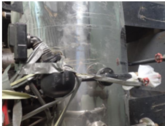
Figure D.36.28 Series 1505J Low Water Cut-Off/Pump Generator
