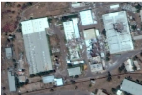
Figure A.60.4 Second strike damage (Post August 2016)
