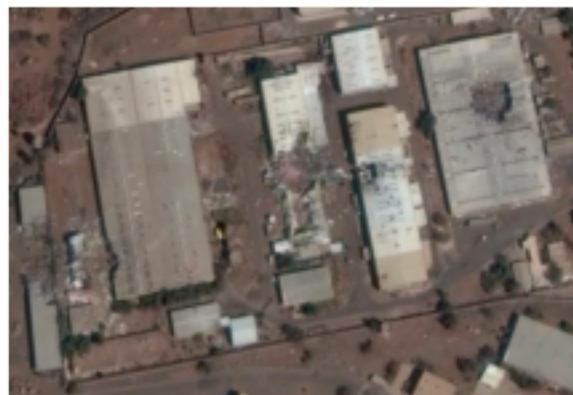
Figure A.60.3 First strike damage (29 February 2016)
